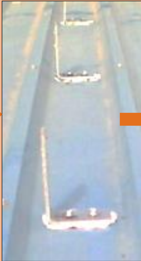
Installation of clamps after penetration and sealing
