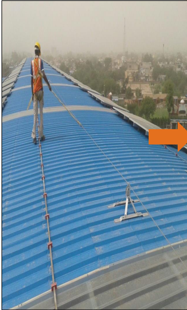
Installation of safety lines
